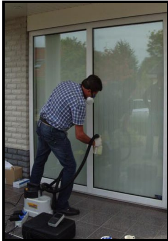
Spraying nano coating on glass Photo courtesy Broekhuizen
