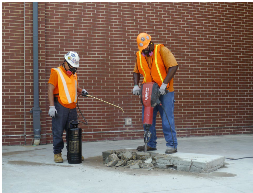
Photo courtesy of the International Masonry Institute & OSHA
