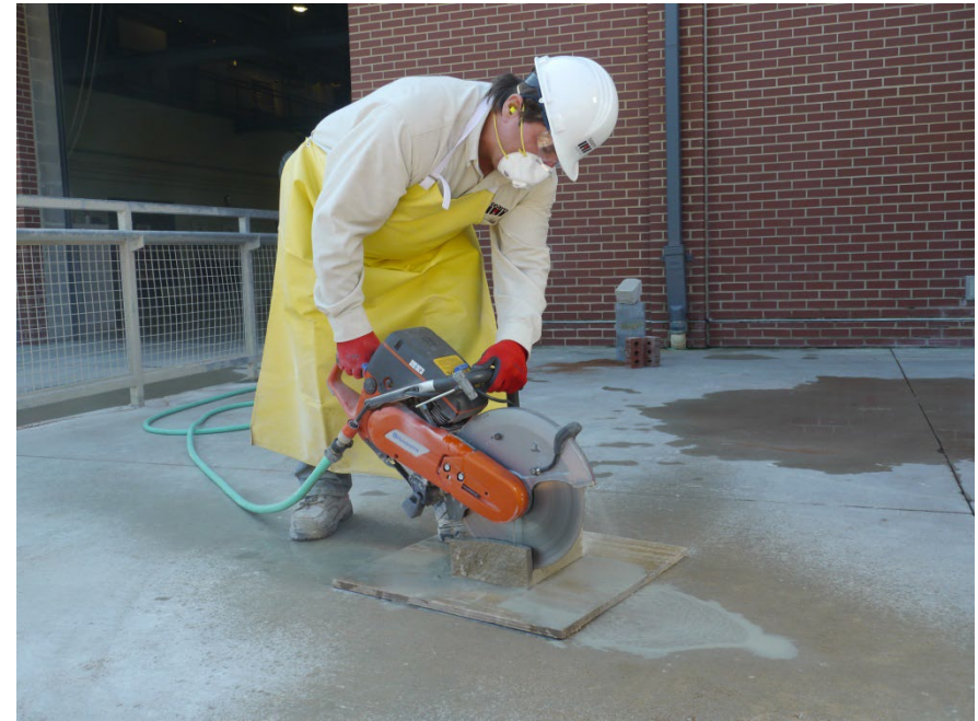
Photo courtesy of the International Masonry Institute & OSHA
