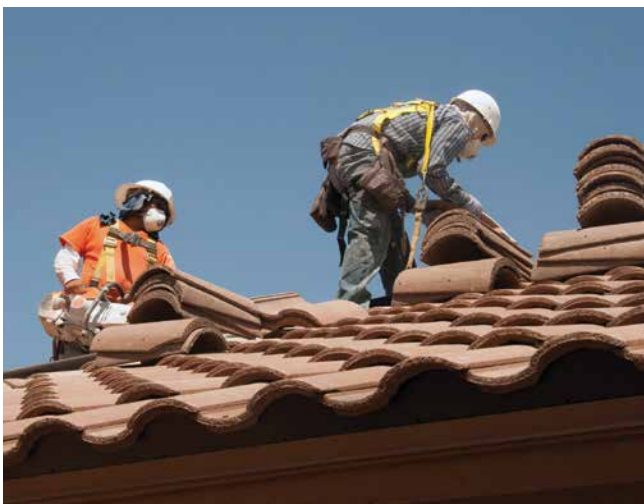
Workers donning fall prevention equipment (Photo courtesy of Wikimedia Commons)
