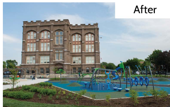
Chicago schoolyard before and after transformation. (Photos courtesy of Justin Brown, MWRD).
