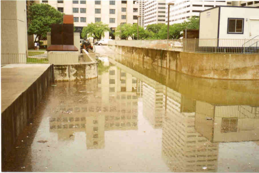
Flooded loading dock before pumping
