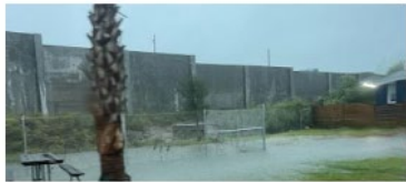
Flooding near the I-26 soundwall at Rosemont, photo by Rosemont residents on September 30, 2022.
