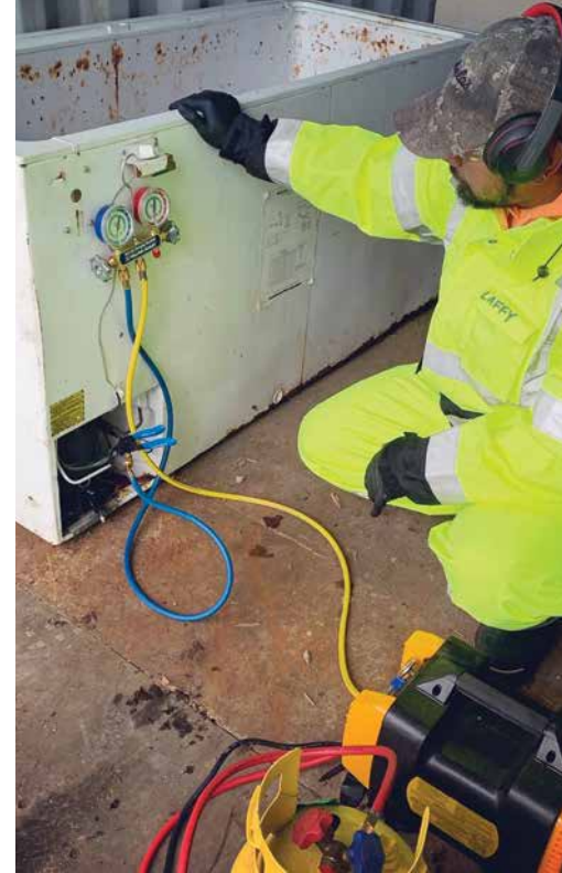
A 2021 RACEJT graduate works in his new job as a refrigerant recovery technician in Kongiganak, Alaska. (Photo courtesy of Zender Environmental)
